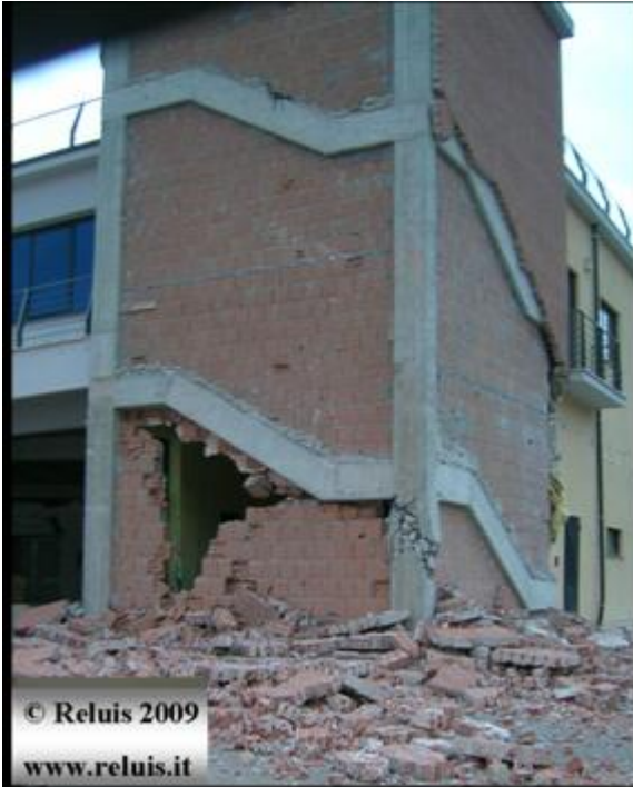
Stairs damage Shear failure of a short column in the staircase. Photo by G. De Carlo and G.M. Verderame
