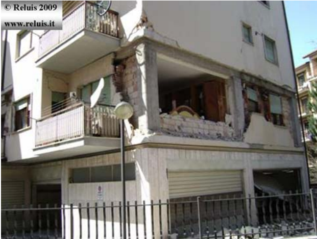
Reinforced concrete building placed in Via XX Settembre – L'Aquila Total and partial ejecting of corner infills at first level. Photo by I. Iervolino
